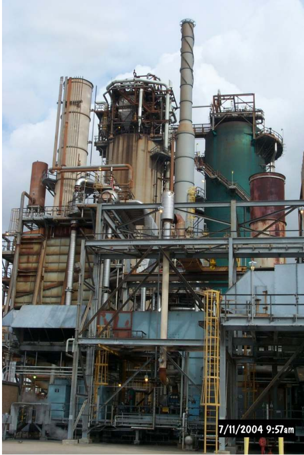
Figure 3. Silo utilizing the FLEXICOKING technology
