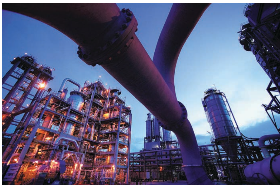
FIG. 3. View of ExxonMobil’s chemical plant in Singapore. The facility is ExxonMobil’s largest integrated manufacturing site in the world. Photo courtesy of ExxonMobil.
